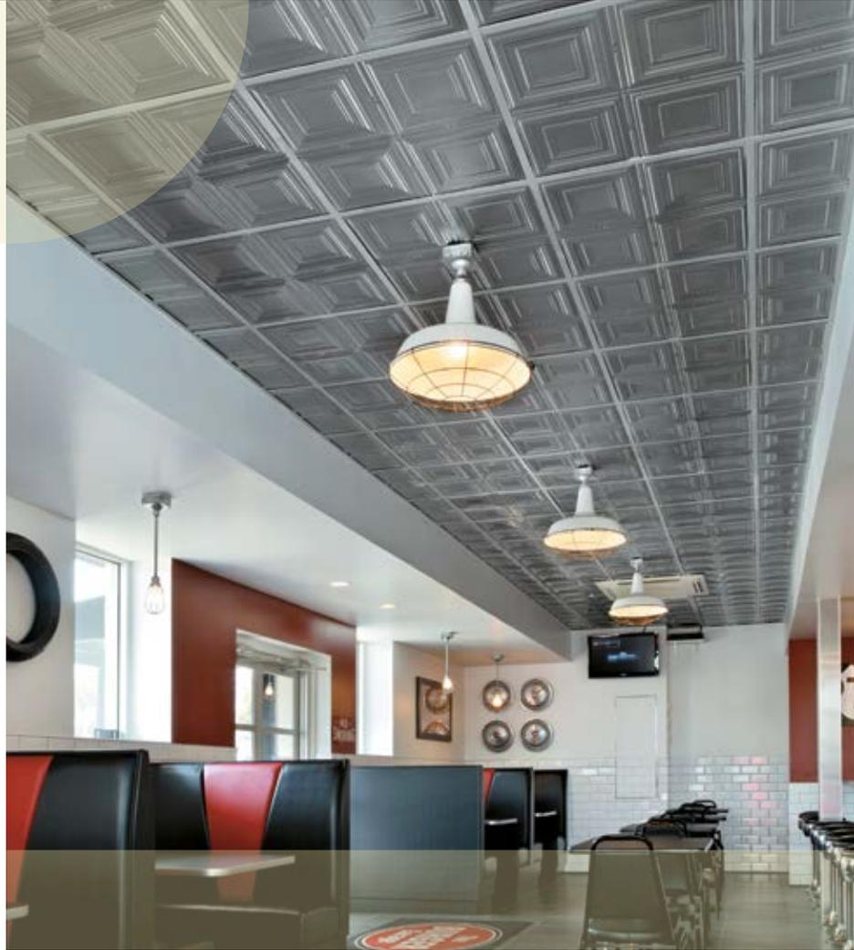
The 2' x 2' Tegular ceiling panels are installed in a 15/16" suspension system in a coordinating color. The combination of the panel reveal edge and the grid color diminishes the overall visibility of the suspension system.
