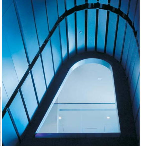
Custom Metal Walls with Rd 1522 perforation and Custom RAL 7024 finish Club Nokia at LA Live!, Los Angeles, CA
