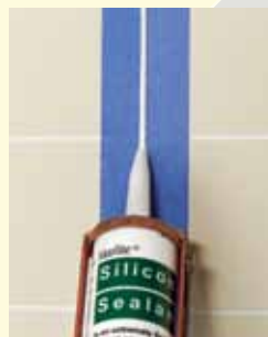
Place a bead of harmonizing Marlite Silicone Sealant in the gap.
