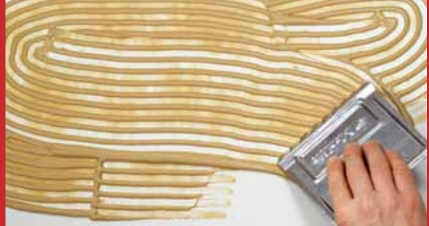
Simply apply Marlite Brand Adhesive to the back of FRP panels and apply them to the subwall.
