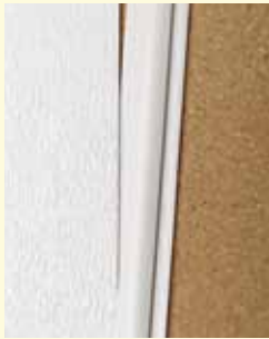
Slide Marlite Division Molding under edge of first panel.
