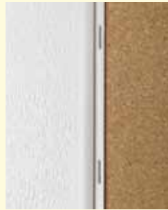
Staple Division Molding to subwall along revealed edge.
