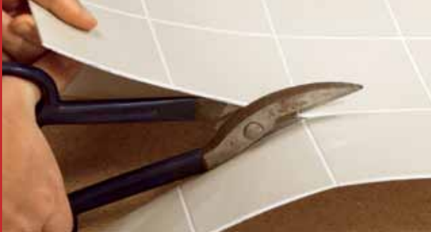
FRP panels can be easily cut with shears or a carbide tip saw.
