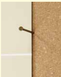
Place a 6 penny spacing nail between panels.
