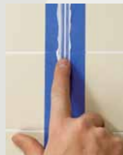
Using your finger, place a slight indentation in the gap.
