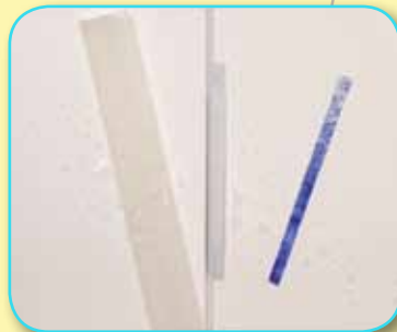
Division trim is removed, revealing dry & white test strip.
